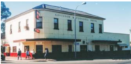
Governor MacDonnell just prior to being demolished in 1996
