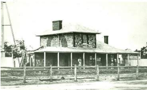
Salisbury Railway Station 1890
